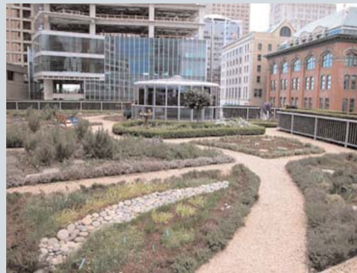
Green roof on the Fairmount Hotel Photo by: David Walker
