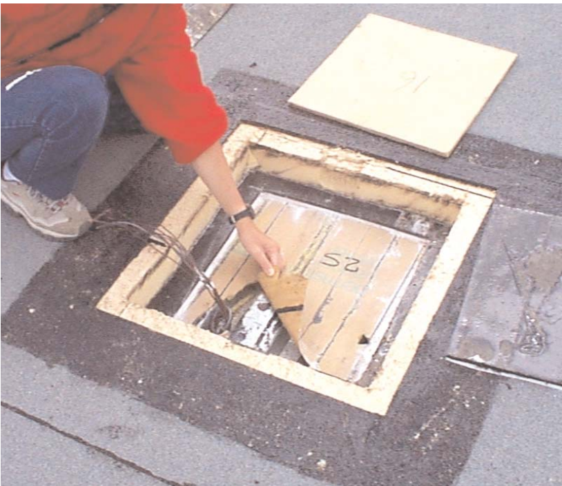
Roof cuts were made on the Eastview Community Centre green roof to allow for sensor installation.
