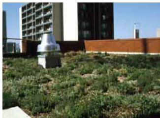
Green Roof System Hamilton Building in Portland, OR
