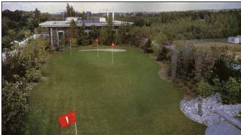
Corporate Golf Course Green Roof
